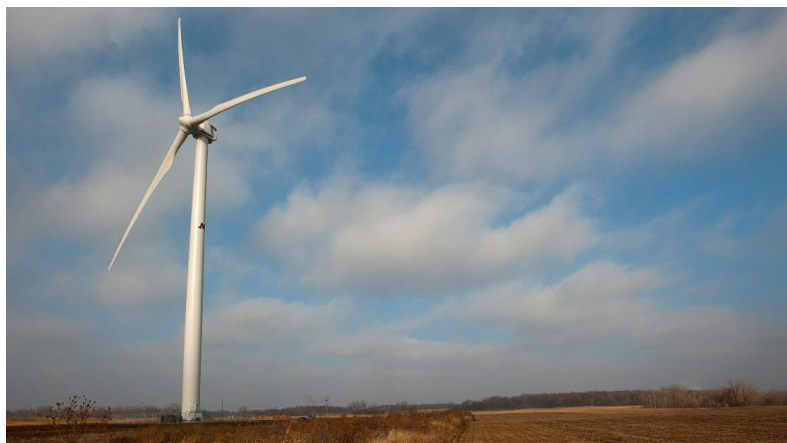
Figure 1. The 2.5 MW Clipper Liberty C96 wind turbine, University of Minnesota
